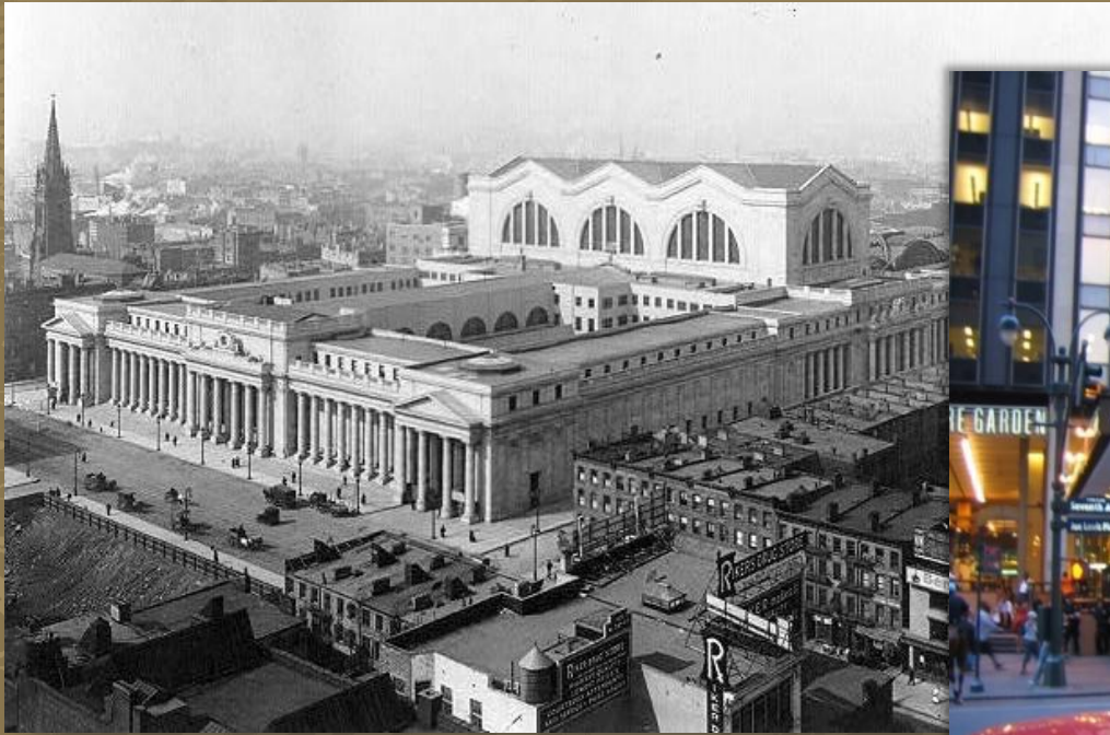
Penn Station, New York before demolition
