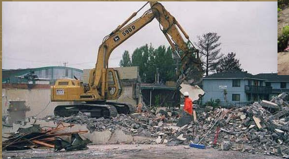
Building demolition, CA
