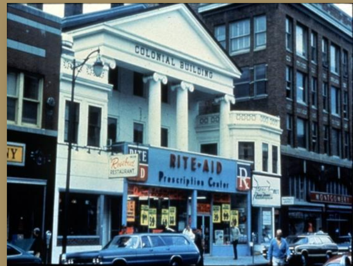
Incompatible addition and use
